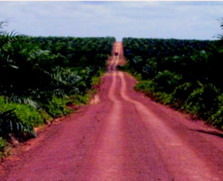
Part of road network
