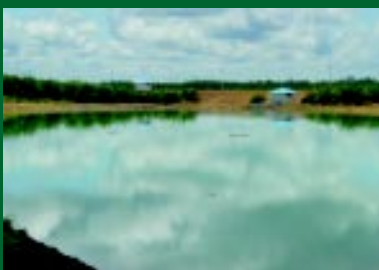
Reservoir - capacity 100,000 cu. mt. (Storage of water for mill consumption)
