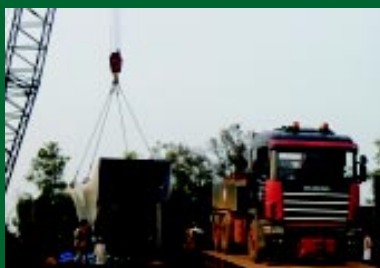
Transportation & unloading boiler
