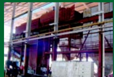
Installation of machinery
