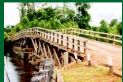
40 metre long bridge
